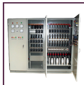
LV CONTROL PANELS & CAPACITOR BANK
